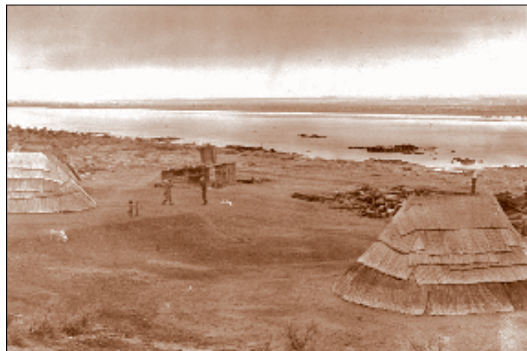
Dwellings made from tule reeds woven into mats were commonly used by Columbia Plateau tribes. This photo shows two Wanapum homes in the 1930s, further down the Columbia River from Rock Island.
