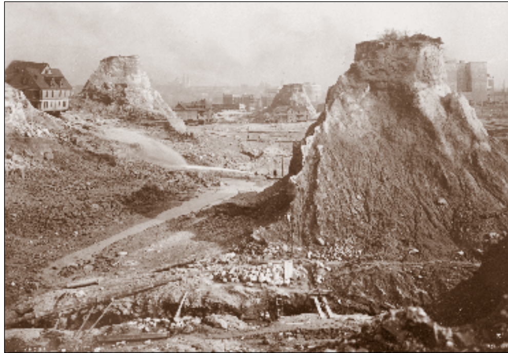
Asahel Curtis captured earth-moving projects as Seattle planners sought to make the city flatter. Some property owners fought the regrades. While their claims were pending in court, contractors sluiced around their land, leaving 50 to 60-foot columns of dirt. This photo of the Denny regrade was taken at 4th and Bell streets in 1910.
