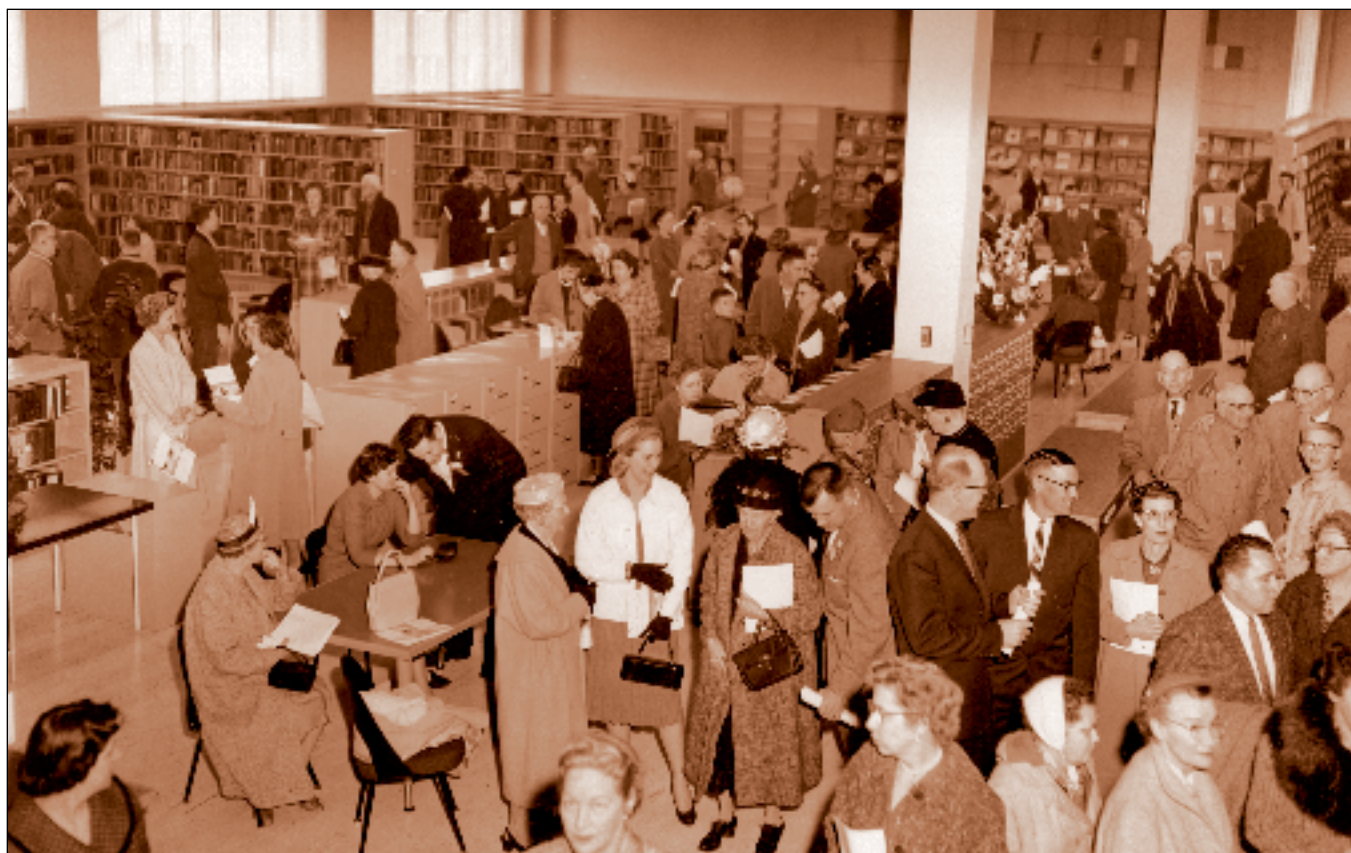
Courtesy of North Central Regional Library
