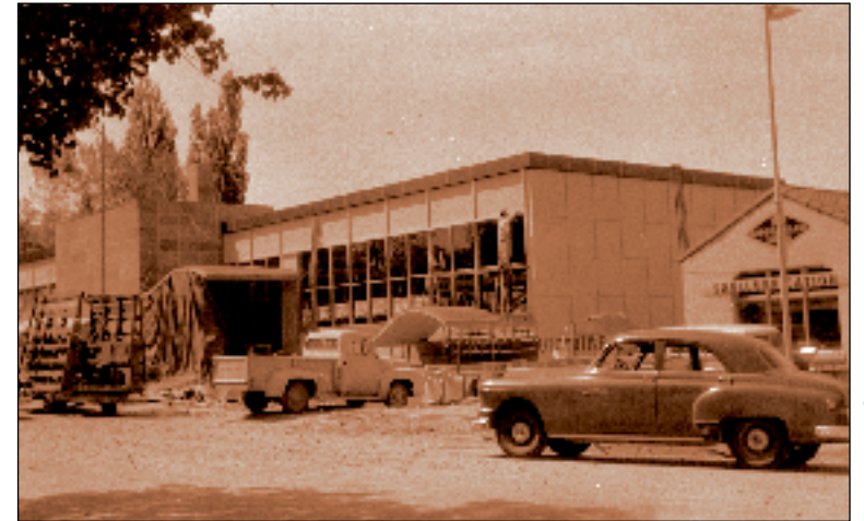
Construction of the new library on Douglas Street was good business for Mack's Shell Station next door.
