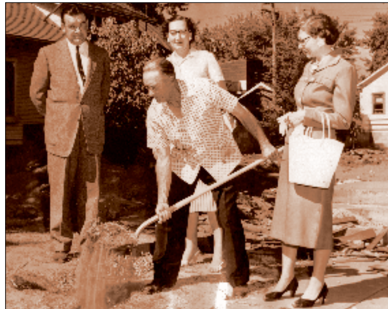
Breaking ground for the new library on Sept. 3, 1957 were, from left, board members Kenneth Graves, Otto Jahns, Kathryn Fewkes and Peggy Ault.
